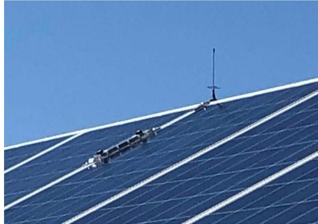
Figure 2: The Deno sensor and antenna mounted in the plane of array between solar modules.
